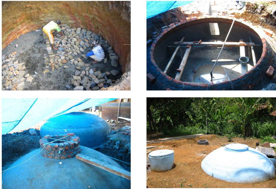
Gambar 2. Disain reaktor biogas tipe fixed dome
